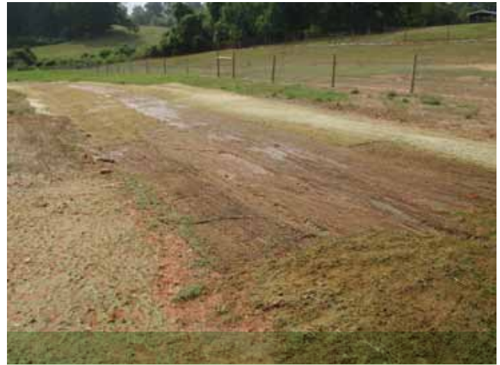
Hydro-seeding reduces water use and promotes fast germination.
