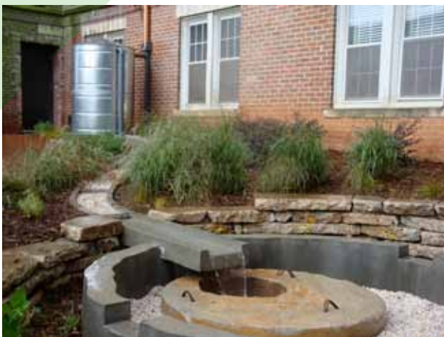
The rain garden at Syme utilizes a cistern to store the collected rain water.
