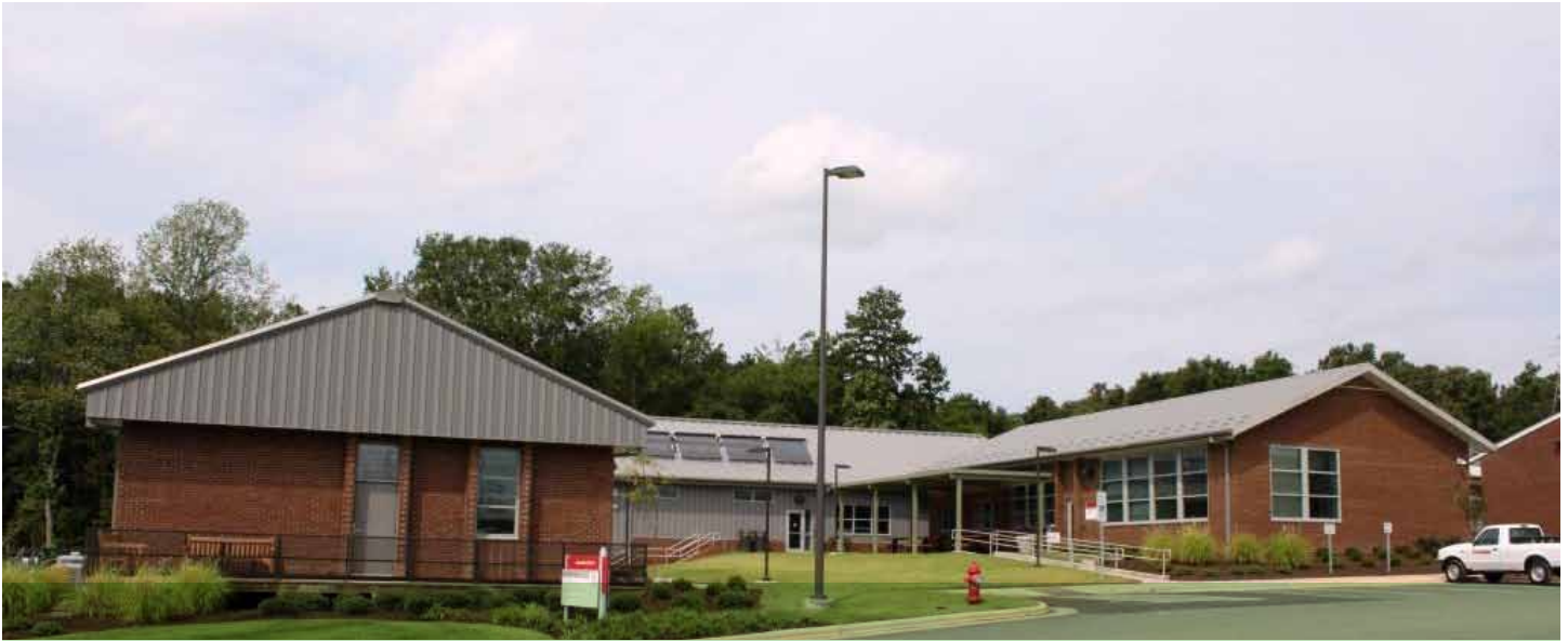
Sullivan Shops III has a solar thermal system on the roof.
