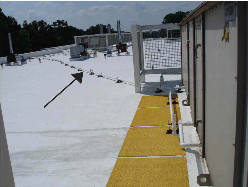
Condensate piping from Air Handling Unit at Flex Building
